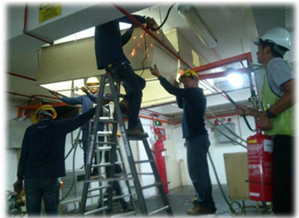
Above: Fire watch during cutting and welding works, vehicle assembly plant. Note the sparks. Batu Kawan, Penang, 2018.
